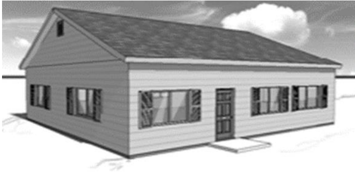
One floor, slab on grade
