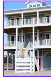
Elevated w/Enclosure on Posts, Pilings or Piers
